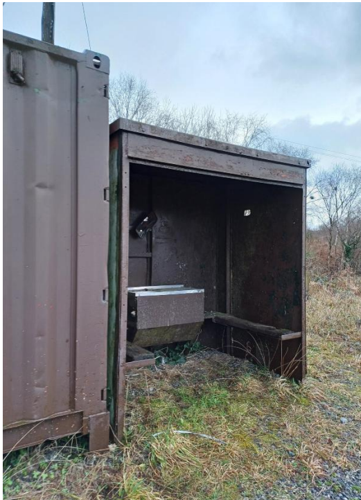
Plate 4-1 – Representative photo of structures within the Application Site – Hand-washing station
